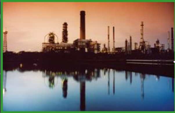
MATHURA REFINERY 8 MMTPA
